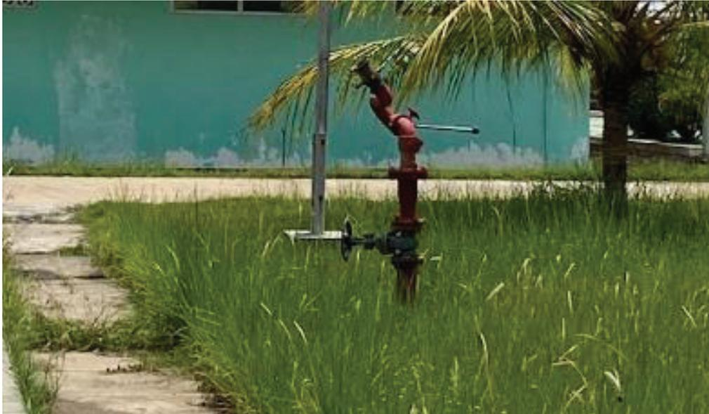
Gambar 4. *Fire monitor nozzle*
