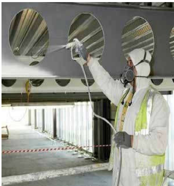
Gambar 7. Application of Intumescent Pain at Construction Site
