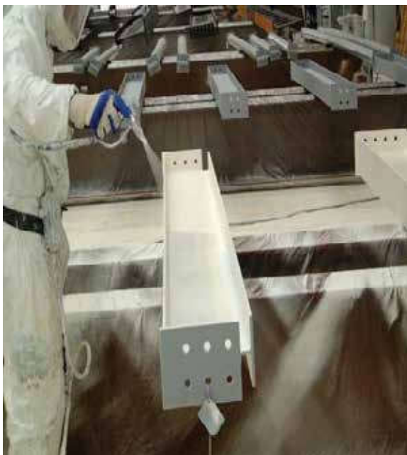
Gambar 6. Intumescent Application Offsite
