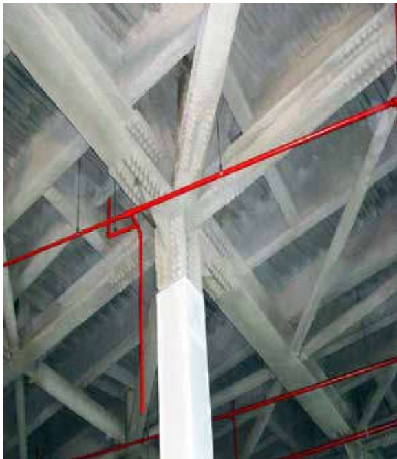
Gambar 5. Concrete Fire Protection System Used for Structural Steel
