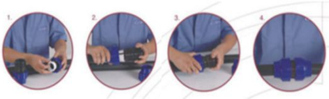
Gambar 6 Metode Compression Fitting
