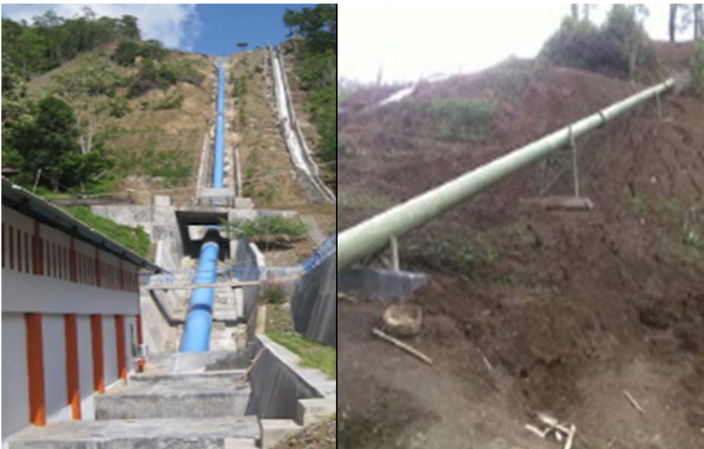
Gambar 8. Pipa Pesat (Penstok)
