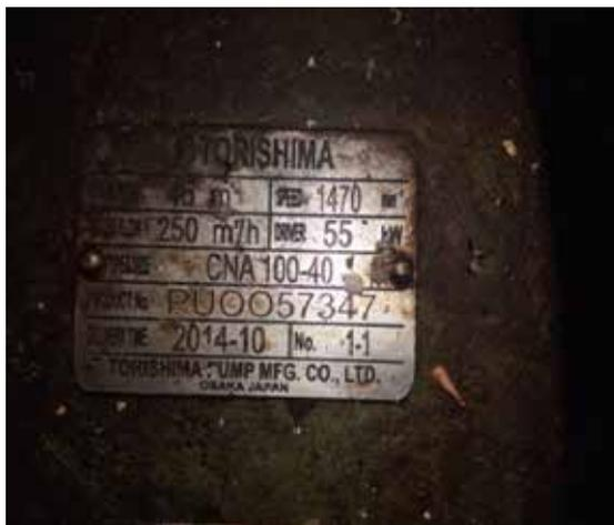
Gambar 6. Name plate Pompa
