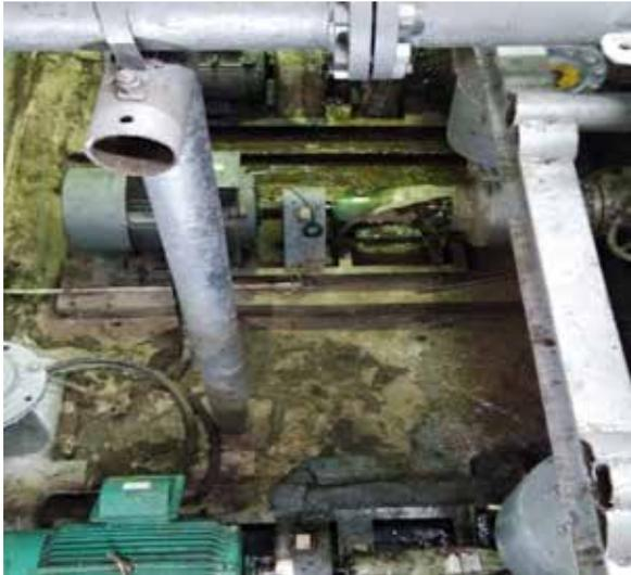
Gambar 10. Kebocoran Pompa Kali Solo I
