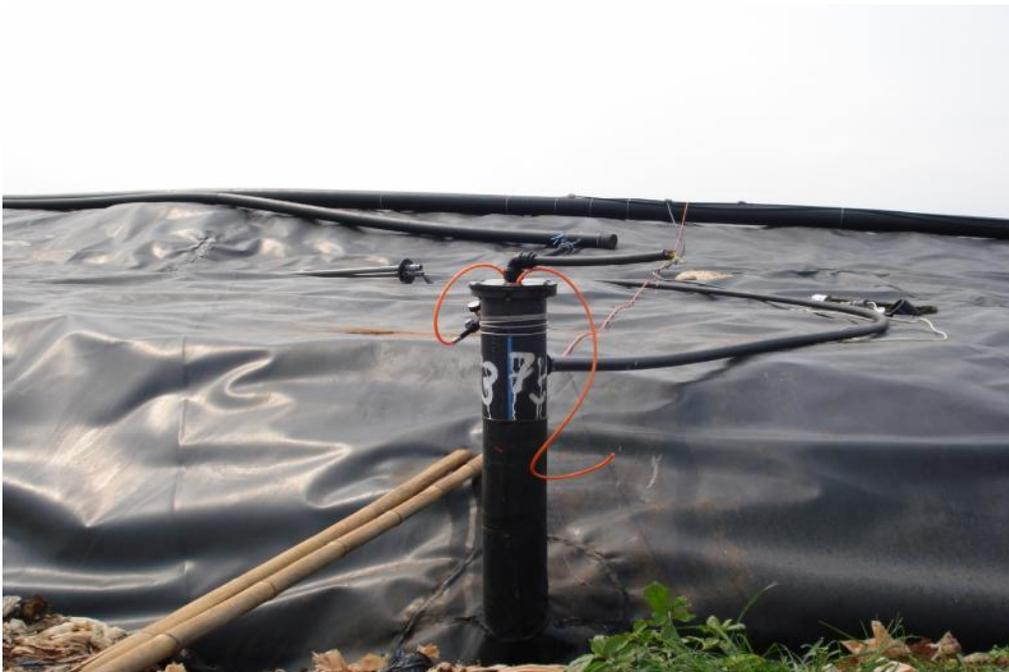
Gambar 6 : Sumur gas methane
