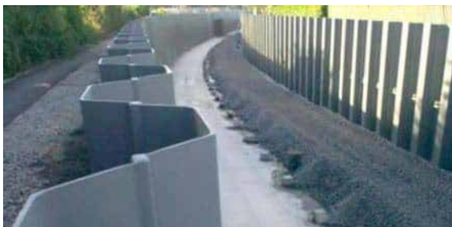
Gambar 16. Sheet pile retaining wall
