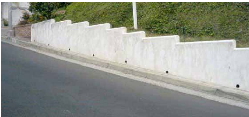
Gambar 19. Weep hole in retaining wall
