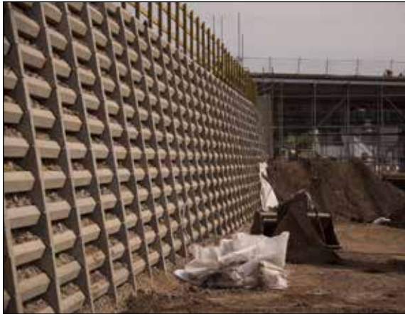
Gambar 4. Crib retaining wall
